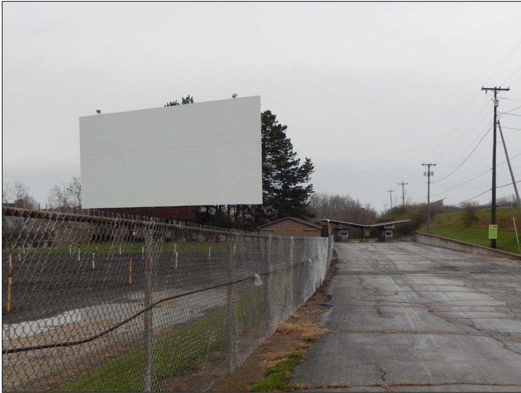
Plate 44. Aut-O-Rama Twin Drive-In Movie Theater (LOR 0231904), constructed in 1965, 33395 Lorain Rd., North Ridgefield.
