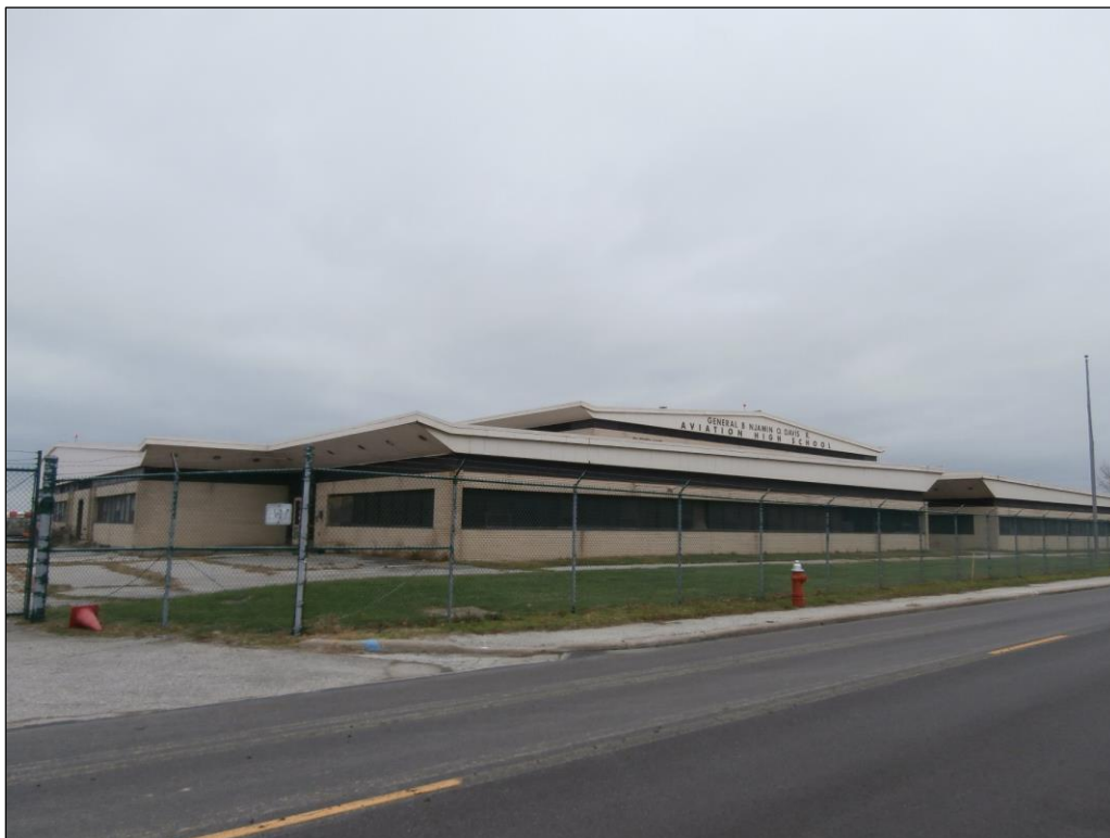
Plate 51. Aviation High School (CUY 1127501), constructed in 1972, N. Marginal Rd., Cleveland.
