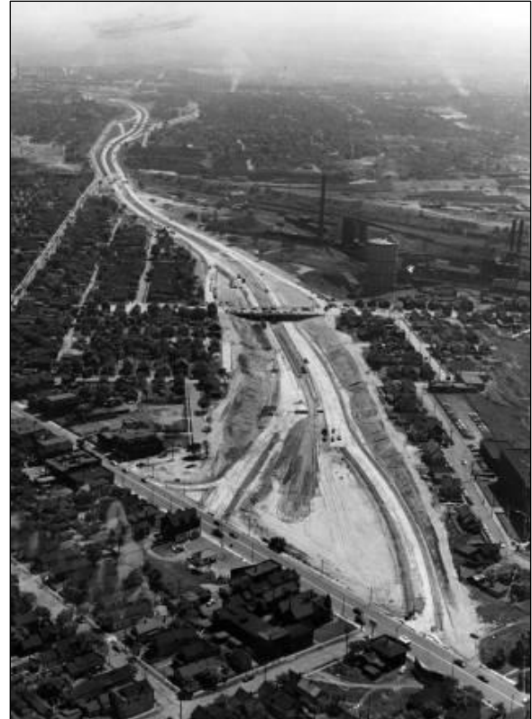
Figure 14-1. 1952 aerial of the construction of Willow Freeway (Cleveland Press Collection, Michael Schwartz Library, Cleveland State University).
