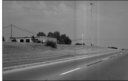
A cell tower in Clark County
