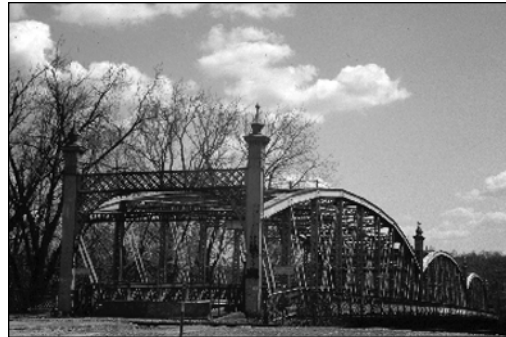
Iron truss bridge in Bridgeport
