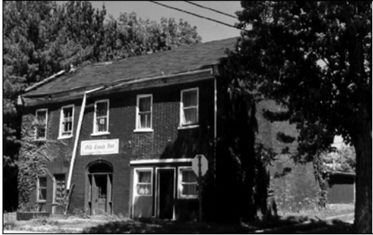
National Road tavern in Brownsville in need of rehabilitation
