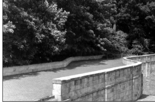
Fox Creek "S" Bridge, New Concord
