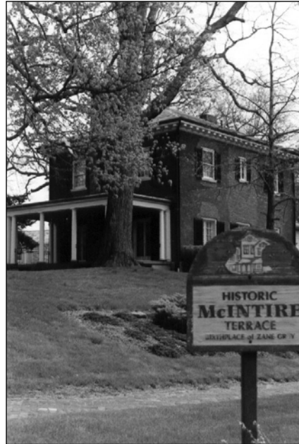
McIntire Terrace, Zanesville – A National Register Historic District
