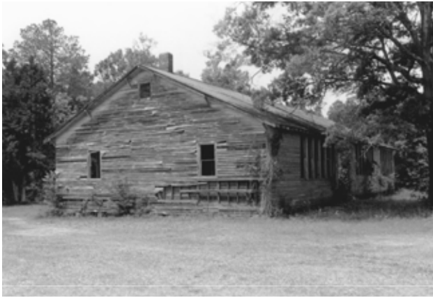
Howard Junior High School, a Rosenwald Fund school built 1924–1925 in Newberry County, South Carolina. National Park Service.
