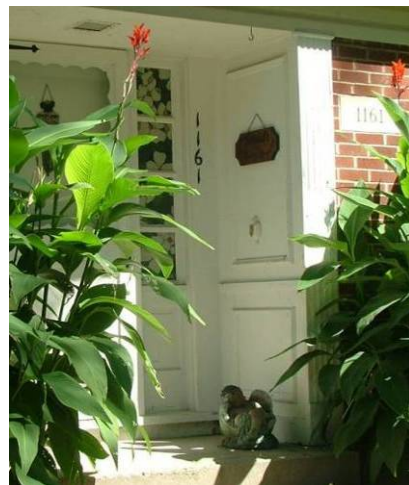
Detail of paneled recessed entry with fluted pilaster 1161 Ashland Ave., Dayton
