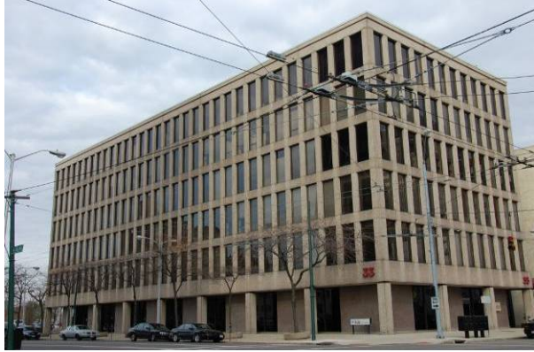
IBM Building 33 W. First St., Dayton
