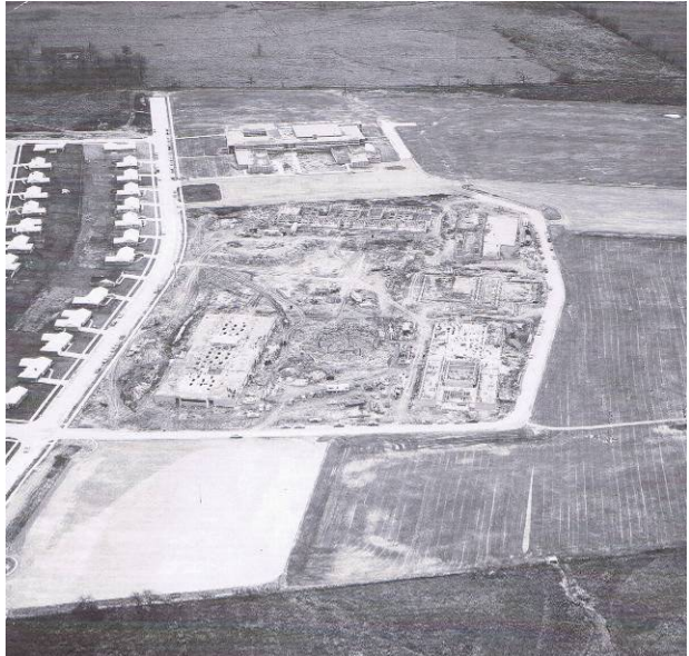
Aerial view, Fairmont East High School under construction, 1962 (Historic Image 42)
