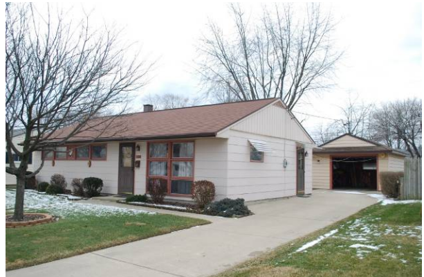
330 North American Blvd., Vandalia
