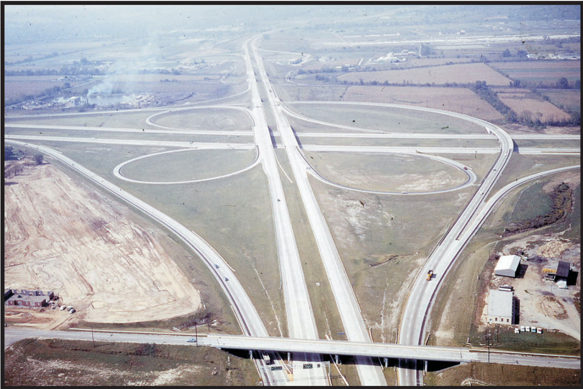
Plate B12. Ca. 1968 view of I-275 and I-75 interchange in Warren County (ODOT Photo Archive 2010d).
