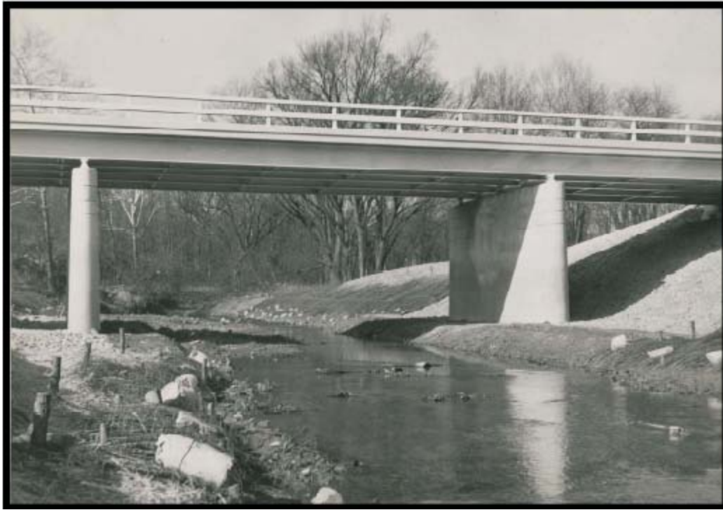
Plate B55. Athens County Bridge in 1961 (ODOT Photo Archive 2010).
