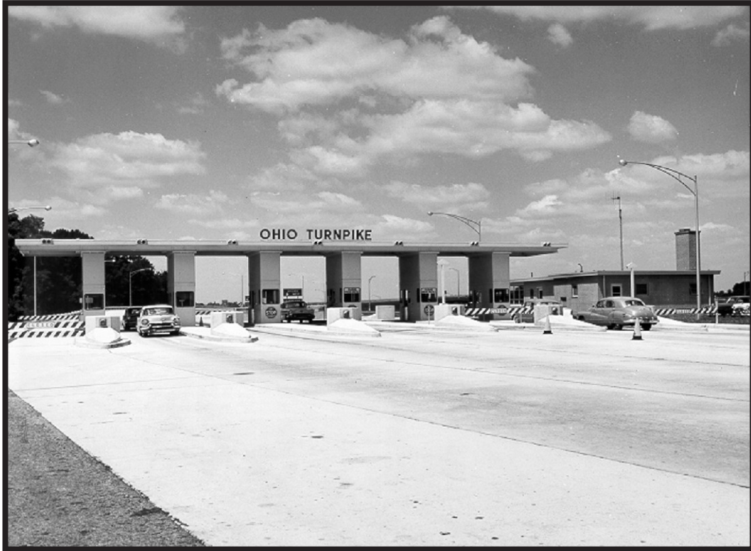
Plate B11. Toll Plaza on Newly Constructed Ohio Turnpike, ca. 1955 (Ohio Turnpike Commission 2007).
