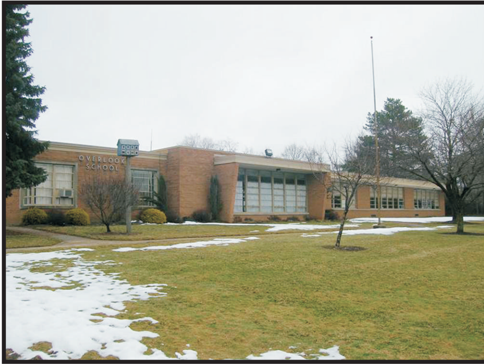
Plate B17. International-style, ca. 1954 Overlook School at 524 Broad Street in Wadsworth, Medina County (Old Ohio Schools 2010).
