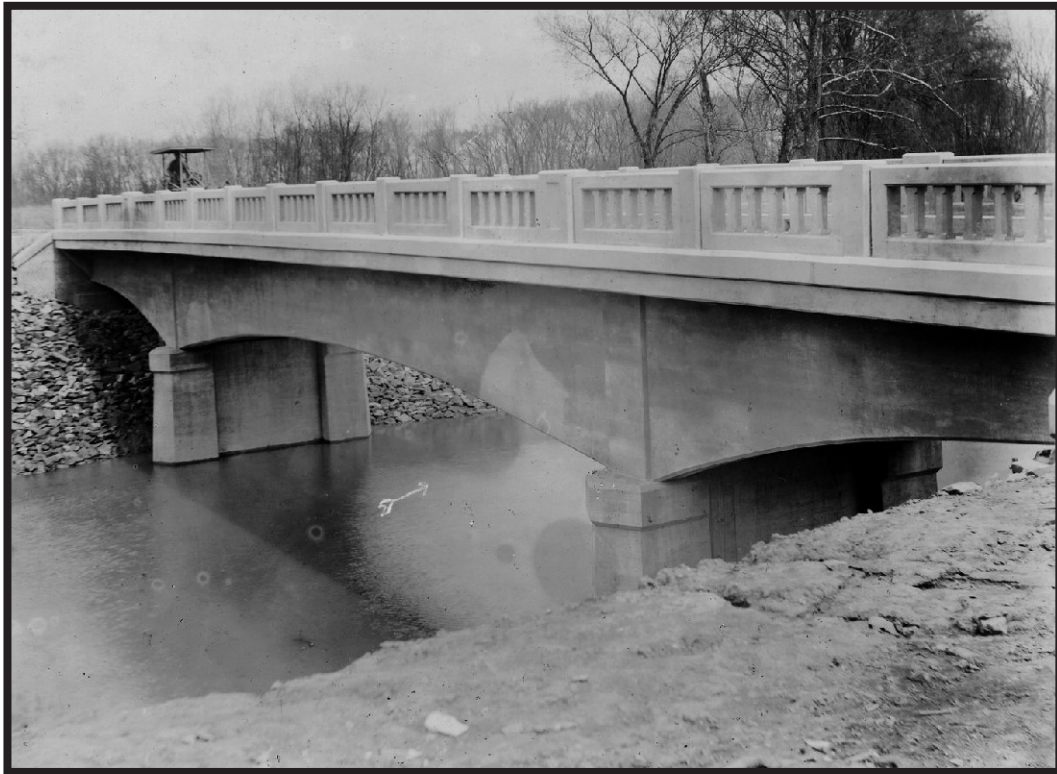
Plate B10. Ca. 1953 view of bridge in Carroll County showing typical design elements and height clearance (ODOT Photo Archive 2010c).
