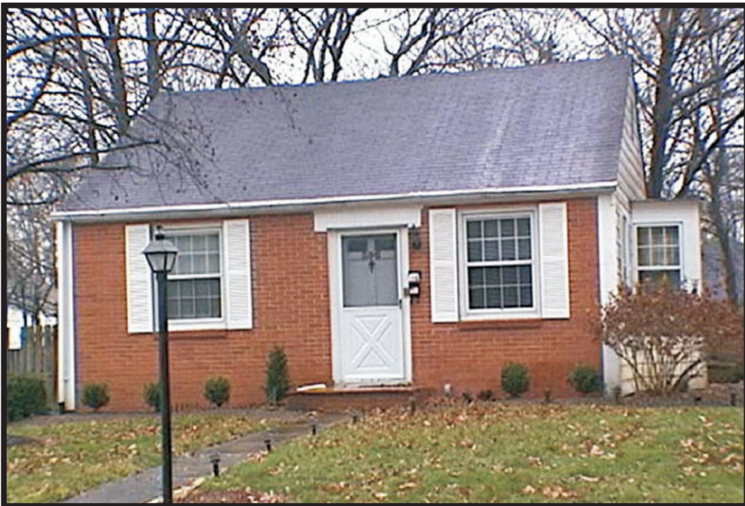
Plate B2. Smallest model house built in Colonial Hills neighborhood in Worthington, ca. 1943 (Campbell 2010a).
