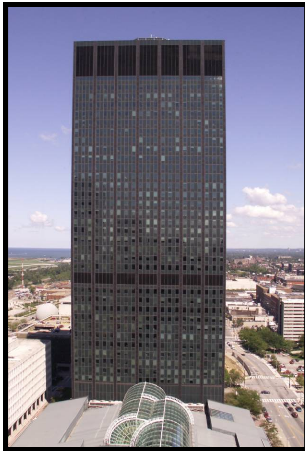
Plate B56. Ca. 1964 Tower at Erieview at 1801 E. 9th Street, an urban renewal project in downtown Cleveland. (Shawn Hoefler, Clevelandskyscrapers.com, 2010)
