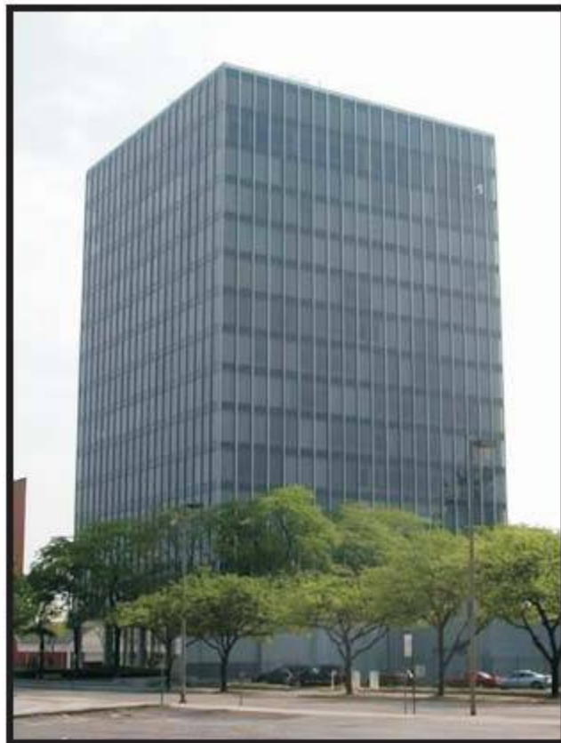
Plate B46. Libbey-Owens-Ford headquarters building, completed in 1960, at 811 Madison Street in downtown Toledo (University of Toledo Libraries Canaday Center 2007a).
