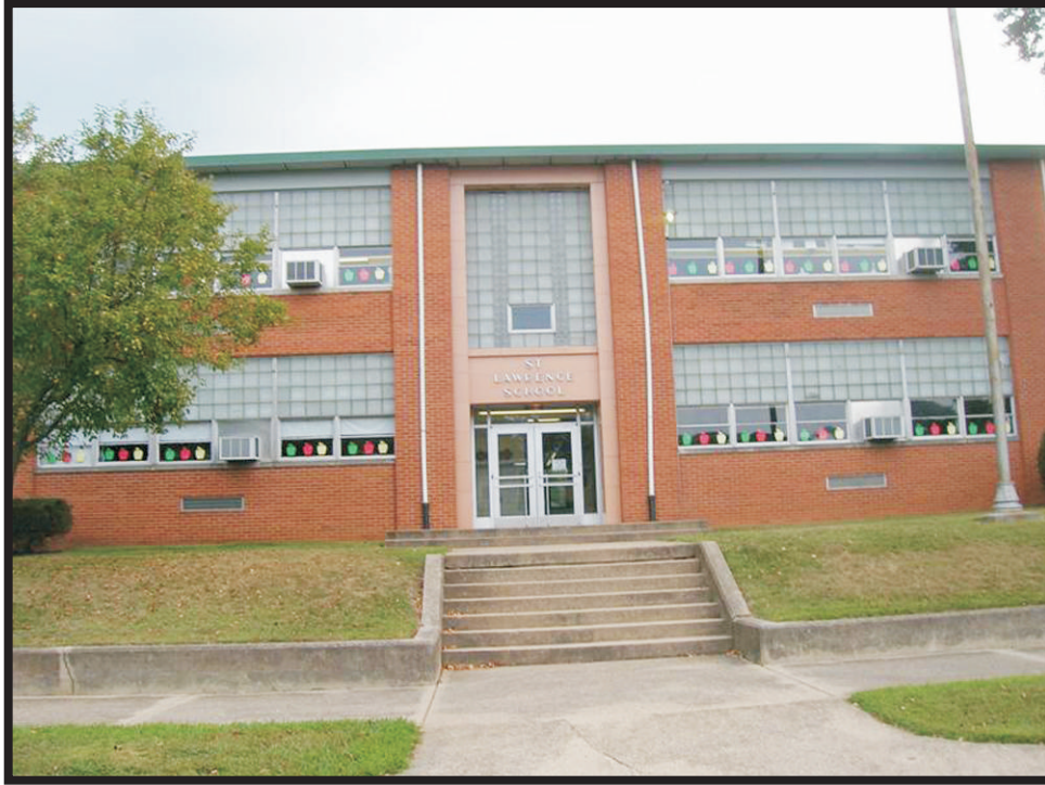
Plate B15. International-style, ca. 1959 Lawrence Street School #2 at N. Seventh Street in Ironton (Old Ohio Schools 2010).
