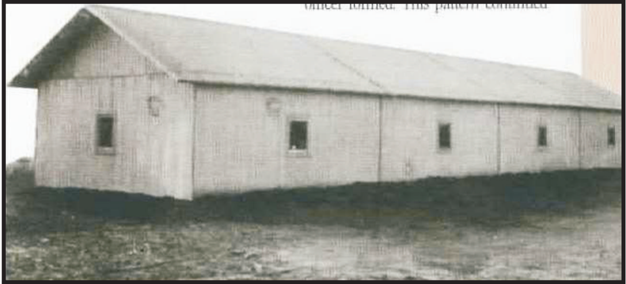
Plate B7. Example of an early model of a prefabricated building designed by the Butler Manufacturing Company (Butler Manufacturing Company n.d.).
