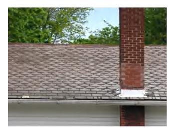
The roof is the first line of defense in the battle to keep water out of a building. This original slate roof has many years of service life left, but it must be cared for properly. The most important things to do are to replace or re-install any missing or dislodged slates; and to avoid walking directly on the roof surface while doing work.
