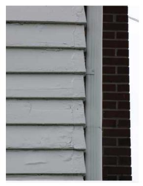
This wood siding, an example of traditional beveled siding, was installed in a way that accentuated the overlap of the boards when viewed from the corner. This was done purposely by the builder as part of the design, to add depth and texture to the building's surface. Especially in cases like this, but on any building that has retained its original siding, replacement siding should be avoided so that such original design effects are not lost.
