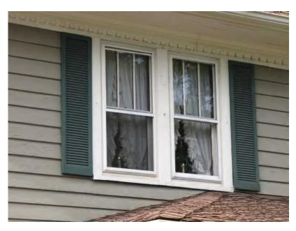
These windows are original to the early 20<sup>th</sup> century house where they are installed. They are "three-over-one" double hung sash windows. They have modern storm windows that have a minimal visual impact, with a dividing bar directly in front of the meeting rail of the window sash.
