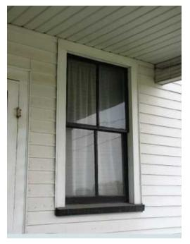
Brookfield is fortunate to have several buildings with original historic wood windows. This is an example of the classic "two-over-two double-hung sash." This means that the upper and lower sash have two glass panes each, and that both sash move independently up and down in slots. In such windows, the upper sash is always offset outside the path of the lower sash.
